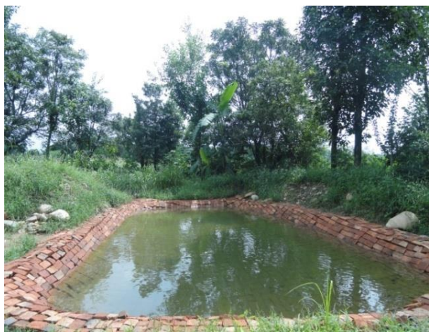
Figure 2: Rain water harvested in polylined tank
