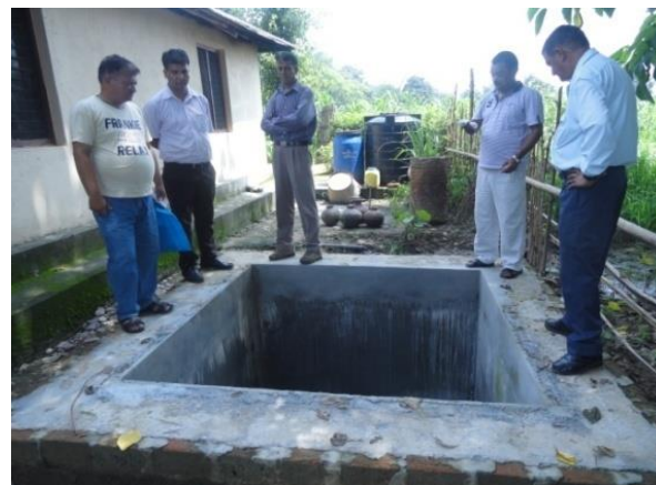
Figure 3: Preparation and demarcation of roof rainwater harvesting tank
