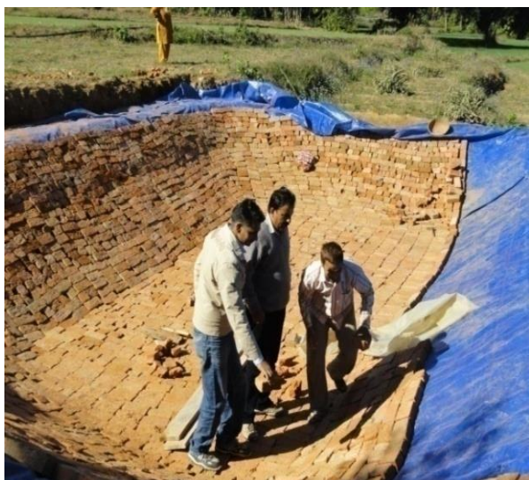
Figure 1: Preparation of polylined tank
